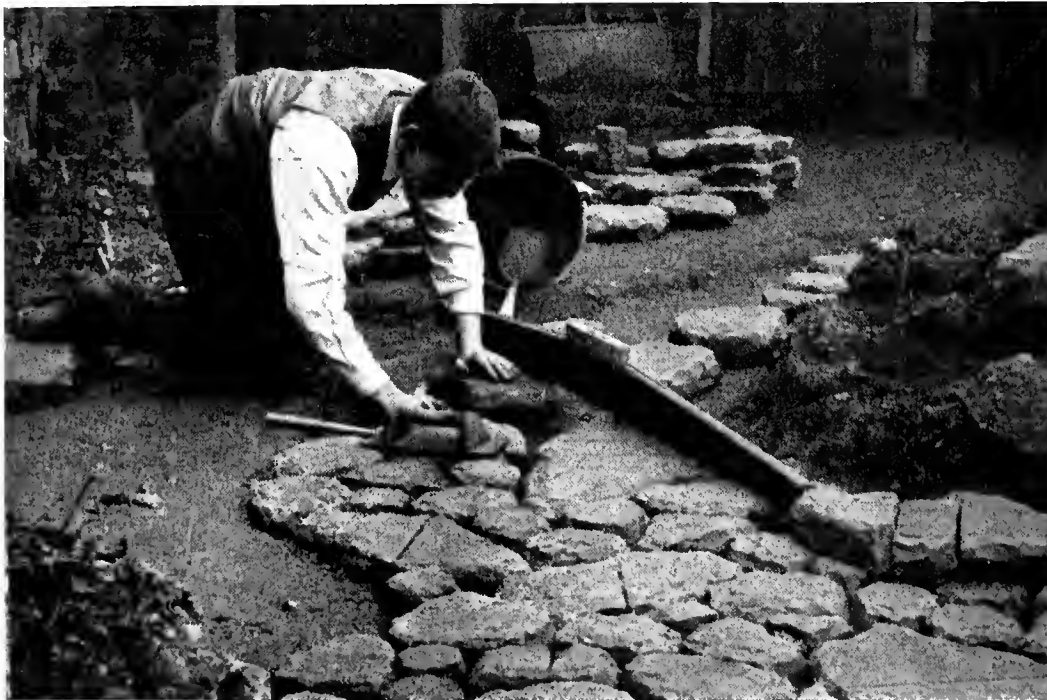
METHOD OF LAYING A STONE PATHWAY. (See opposite page.)
